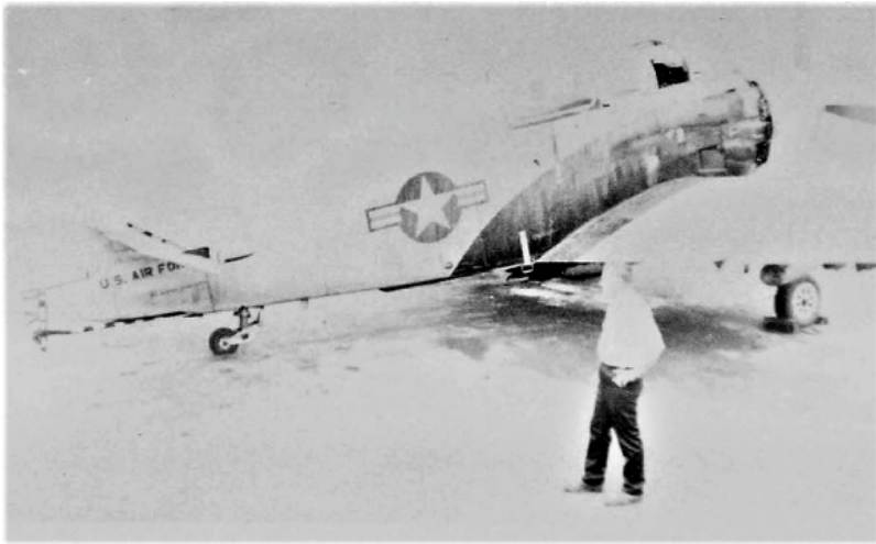
A-1G Skyraider of the 1st Air Commando Squadron, rebuilt by the 633D Consolidated Aircraft Maintenance Squadron with parts from nine aircraft, 8 Jun 1966, 1,576 hours. (633 ABW/HO Archive).
